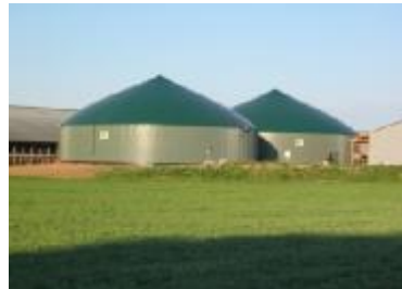
Anaerobic Digester 厌氧发酵
